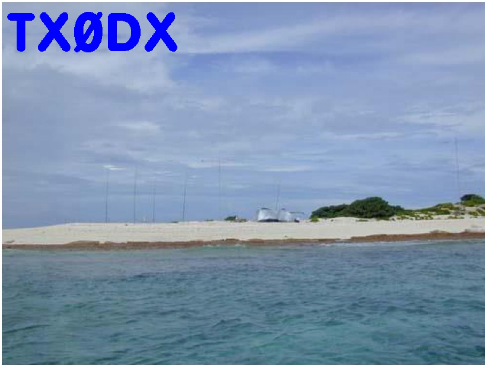
Main antennas on N-S line to eliminate qrm from other site. Main beam directions are 330 and 50 degrees (EU and US) Verticals near the sea.
